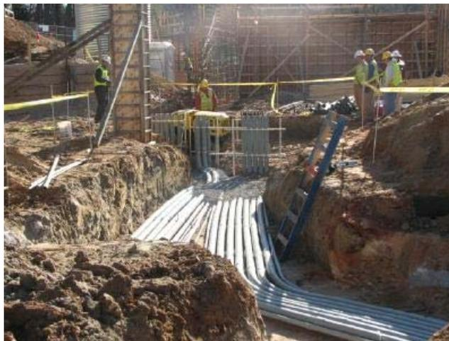
**Figure 1** Underground utility building feeds.
